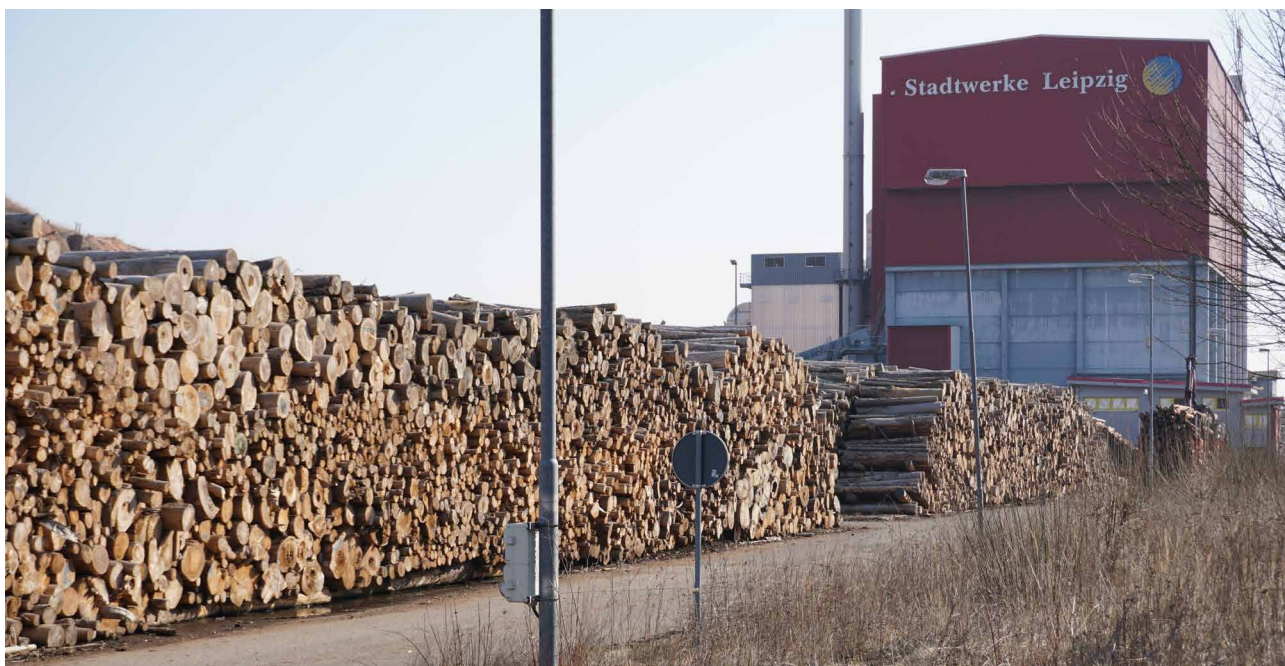
Biomassekraftwerk (biomass power plant) Bischofferode receives EEG biomass subsidies. Photo Credit: Jana Ballenthien, Robin Wood
